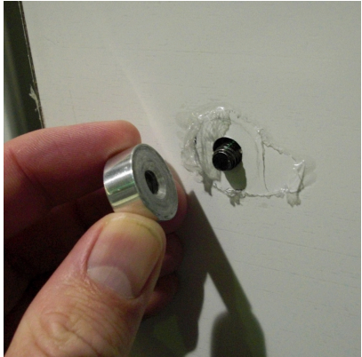
Place lightbox onto the studs in the grooves of the M1020. Secure in place with 3/4" polished standoff caps, 4 per lightbox.
